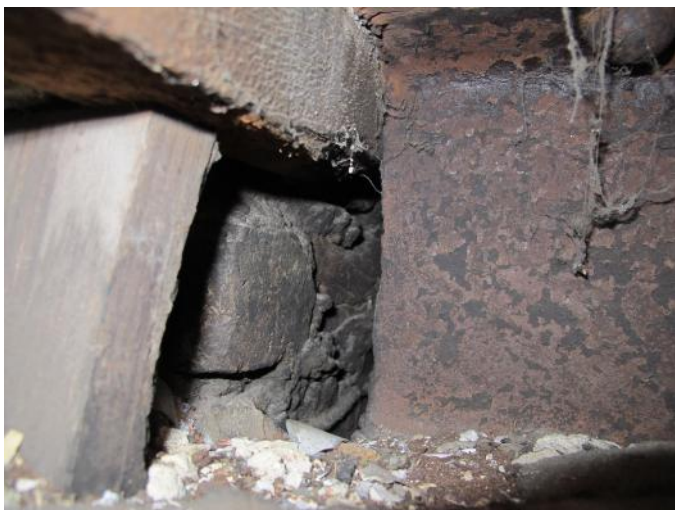
10. The George & Dragon opening to inspect wrought iron beam - view showing no connectivity to party wall masonry
