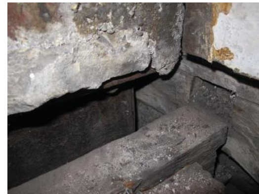
2. Opening up of timber joint between floor trimmer and beam below flank wall
