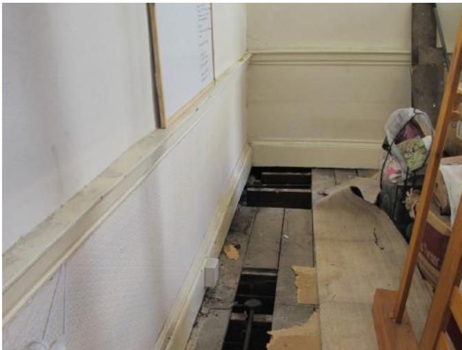
19. The George & Dragon opening to inspect floor structure at spine wall junction with Greenwell elevation
