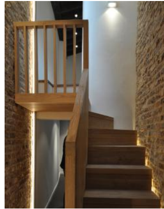
20. New stair and repaired brick work.
