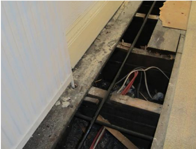
16. The George & Dragon opening to inspect floor structure at spine wall - showing several firings installed to raise the floor level
