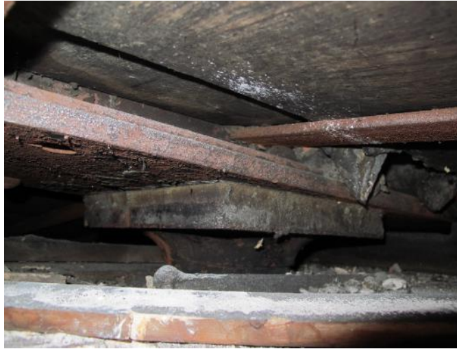
05. The George & Dragon opening to inspect the gable column - view of column head & beam resting on top with no connection
