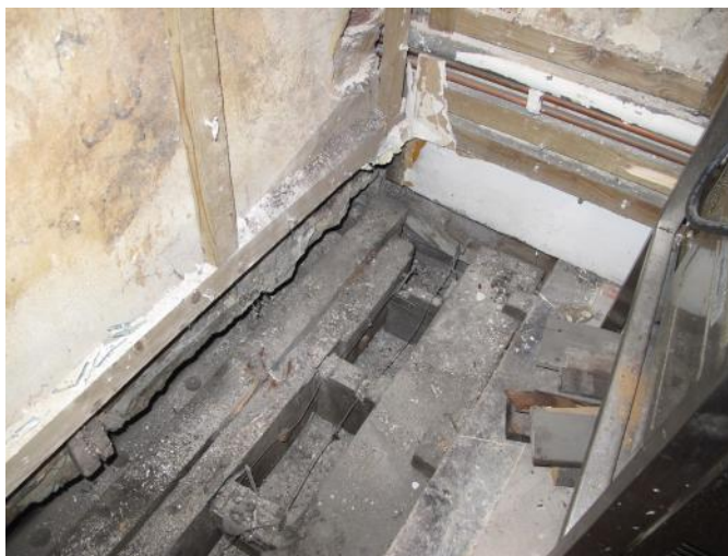
11. The George & Dragon opening to inspect connectivity with wrought iron beam at corner of gable and Greenwell elevation
