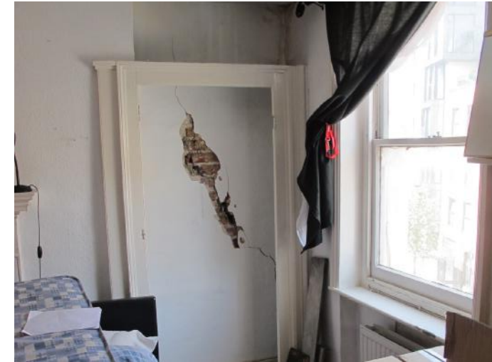
24. The George & Dragon opening to inspect cracking to gable wall at second floor
