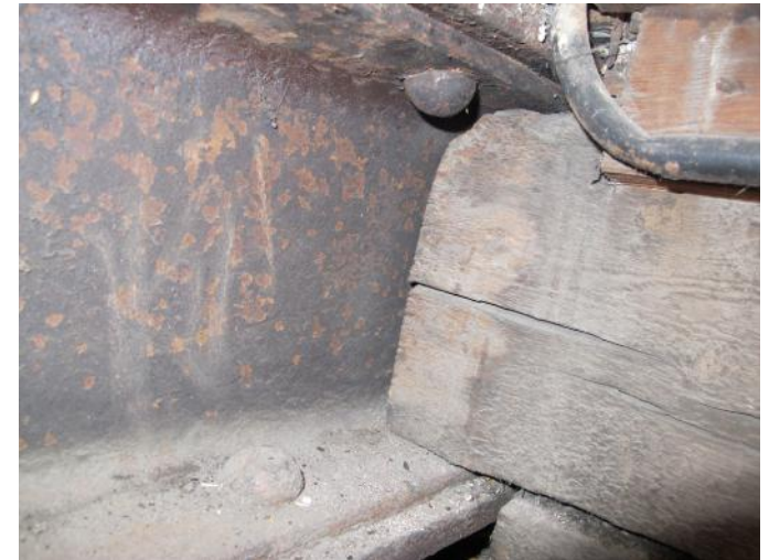
09. The George & Dragon opening to inspect beam - view of floor joist resting on beam
