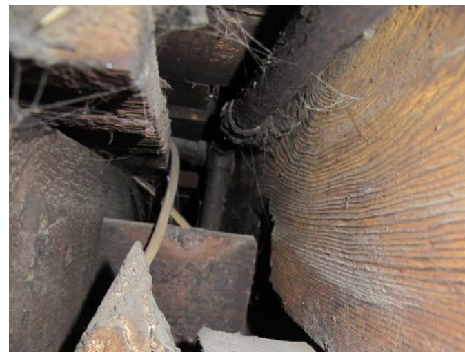
12. The George & Dragon opening to inspect wrought iron beam - view of floor structure unconnected and left hanging
