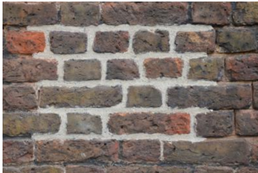
16. Initial repointing mortar joint profile sample panel
