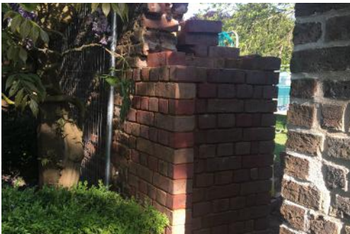
14. The new pier is constructed, toothed into the south wall
