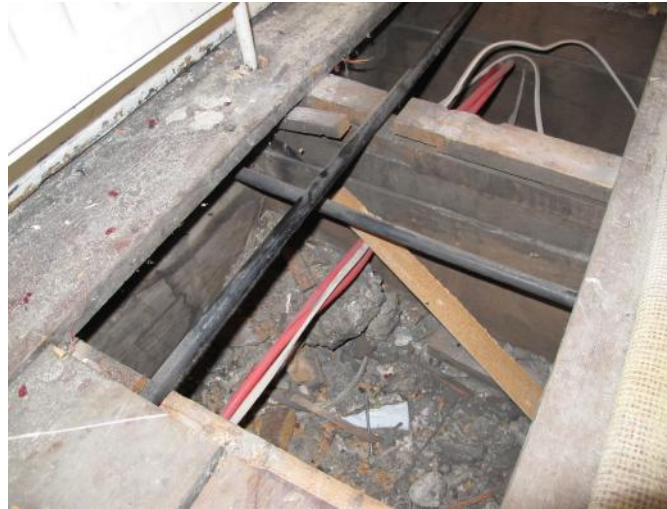
17. The George & Dragon opening to inspect floor structure at spine wall - showing several firings installed to raise the floor level
