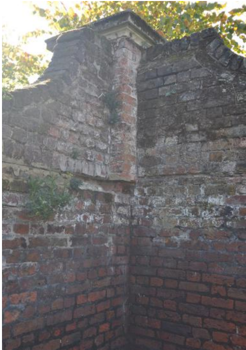
08. Examples of the extent of the damage including crumbling and missing bricks.
