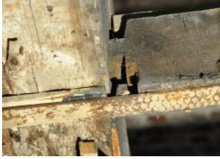
19. Joists dislodged from main beam
