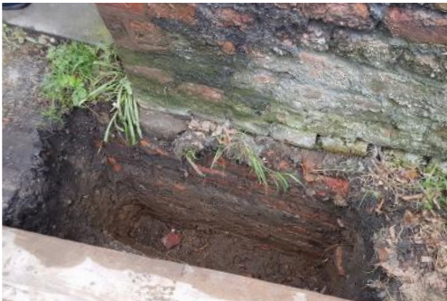
12. Trial pit reveals 8 courses of brick foundation to the south wall
