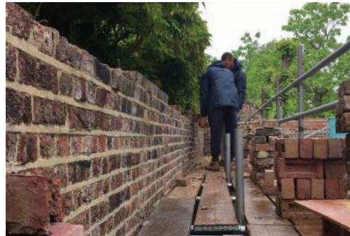
13. The south wall's top four brick courses are removed
