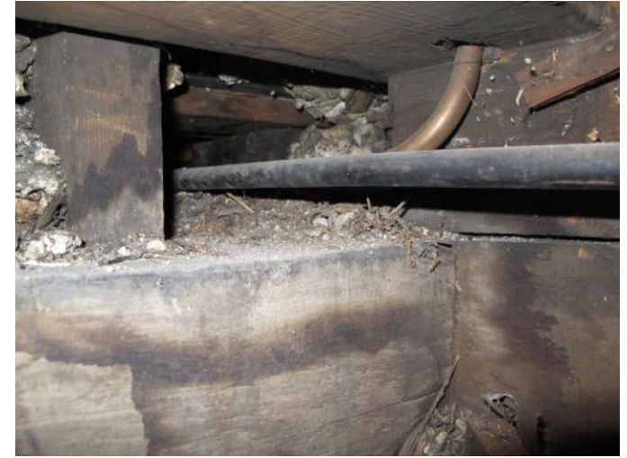
18. The George & Dragon opening to inspect floor structure - view showing spine wall stud resting on a timber beam
