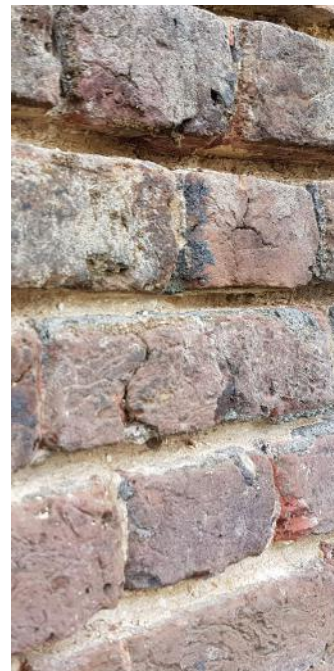
19. Left: bricks raked out to 25mm depth
