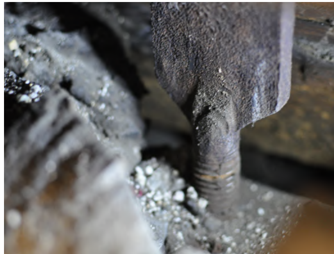
20. The George & Dragon opening to inspect spine wall - view of cast iron structural hanger to the ring beam
