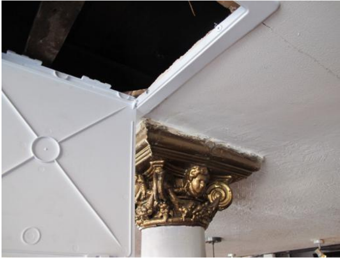
04. The George & Dragon opening to inspect the gable column - location view
