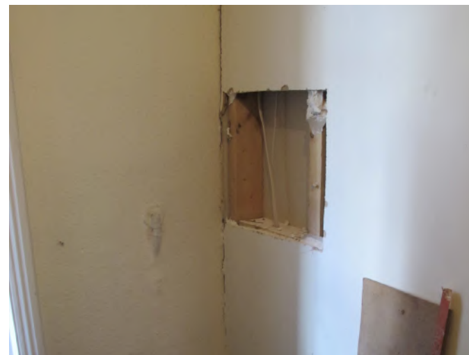
15. The George & Dragon opening to inspect non original partition at first floor - view showing modern studs and plasterboard
