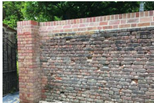
15. The top course of brick, chamfer detail and brick on edge, all in new brick, consolidate the south wall prior to repointing of the existing
