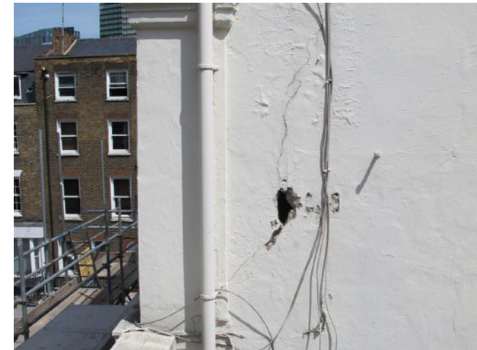
27. The George & Dragon opening to inspect gable wall - view of pronounced cracking to masonry externally
