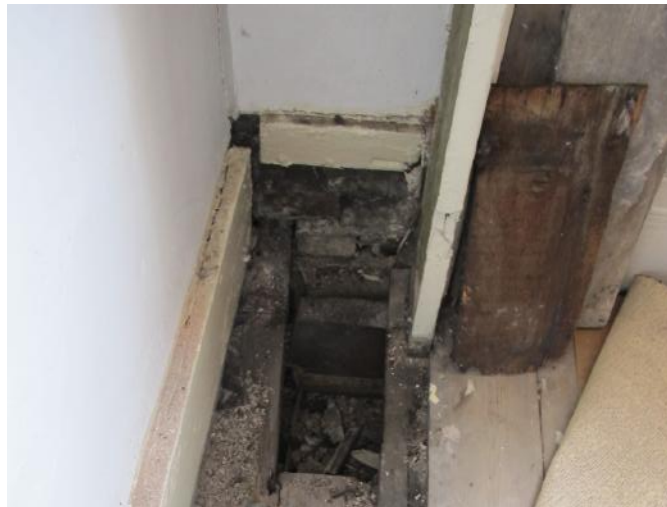
26. The George & Dragon opening to inspect gable wall - view showing no connectivity at second floor level
