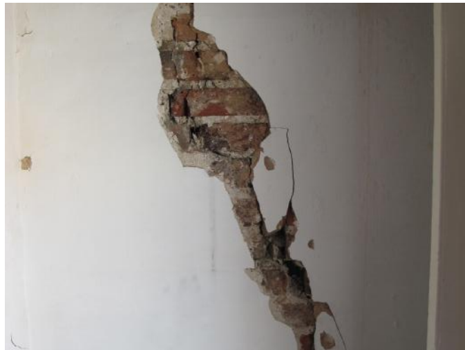
25. The George & Dragon opening to inspect gable wall - view of pronounced cracking to masonry internally
