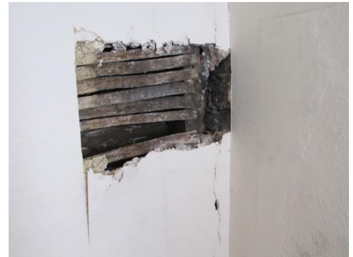
21. The George & Dragon opening to inspect spine wall - view showing original stud and lath and plaster
