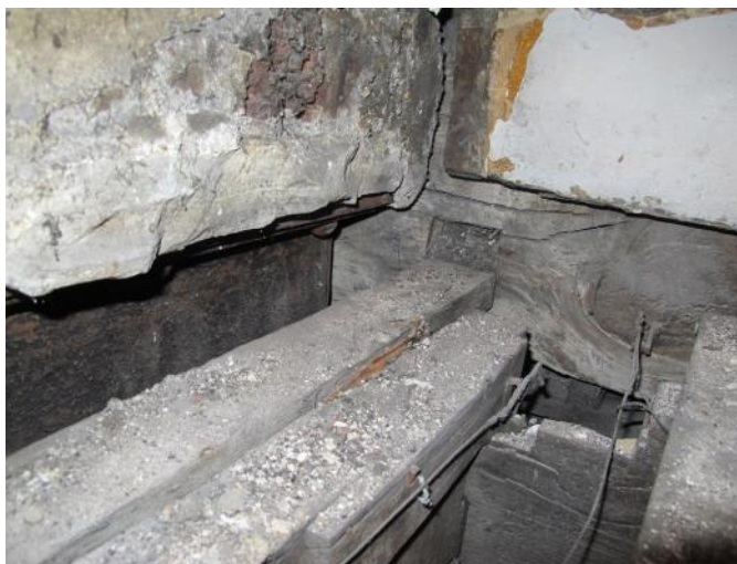
14. The George & Dragon opening to inspect wrought iron beam - view of floor joist mortice having fallen out of its tenon
