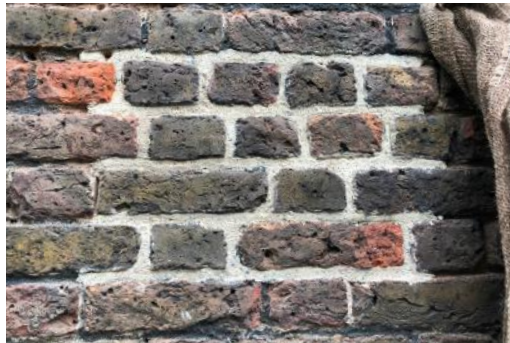
17. Agreed mortar joint profile sample panel, with mortar taken back a further 2mm from face
